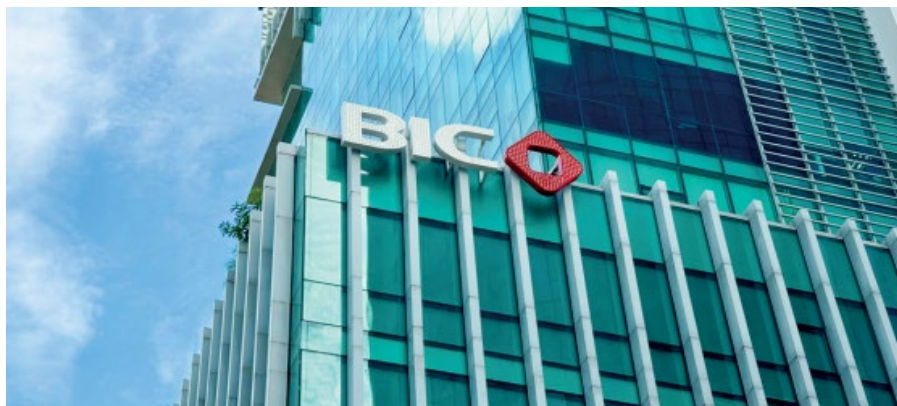
BIC headquarters in Hanoi
