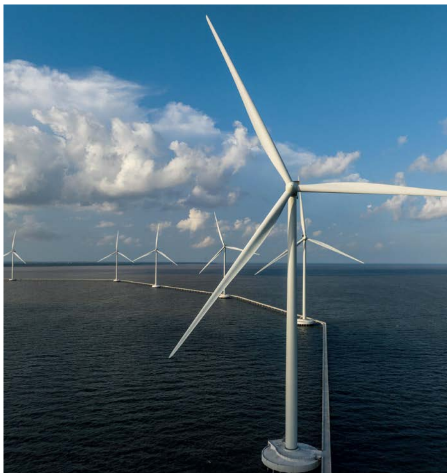
Soc Trang 7 wind power plant financed by BIDV.
